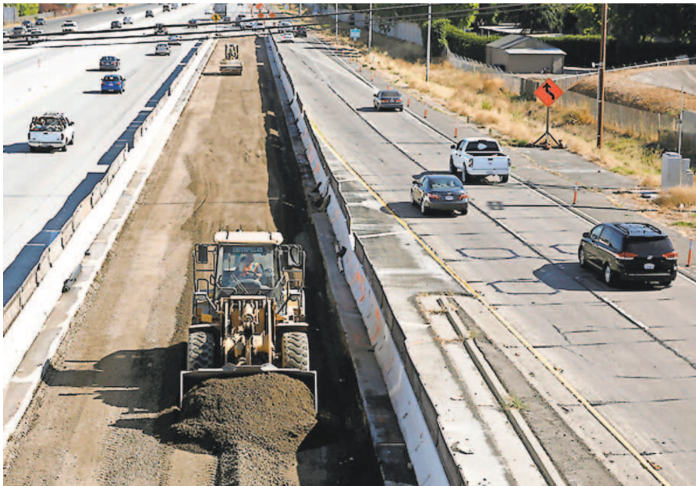
When the bulk of road construction is financed by taxes on gasoline, what happens when electric vehicles become widespread? That’s one issue transportation planners are struggling with. 2015 PHOTO BY RICH PEDRONCELLI, AP
